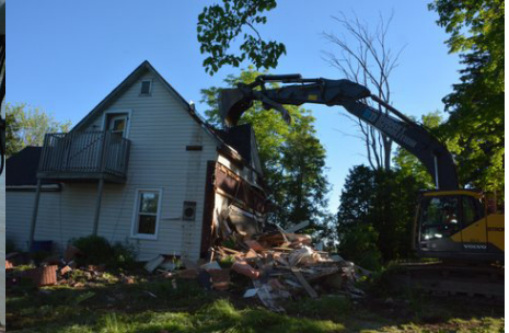
Old Park house being torn down
